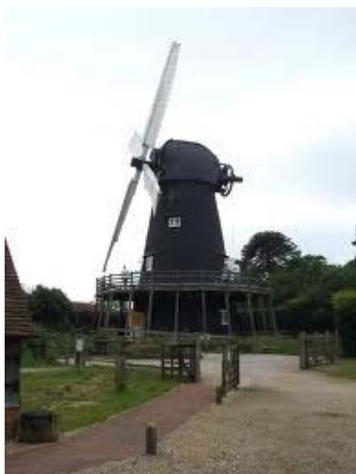
This is done by a simple manually operated mechanism known as a endless chain gear where as most surviving English tower mills have a fantail which automatically keeps the sails facing into the wind. Around the first floor level of the windmill is the reefing stage which is a control platform accessed from the millstone floor level. From here the miller would be able to access the sails from the reefing stage and also operate the endless chain gear and pull the brake rope.
