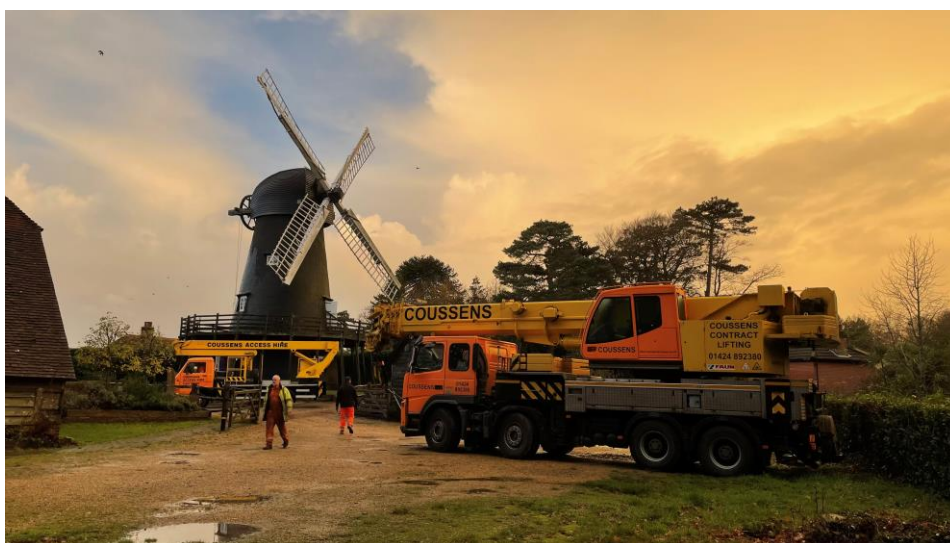
Figure 1 Equipment on site ready for the removal of the stocks and sails
